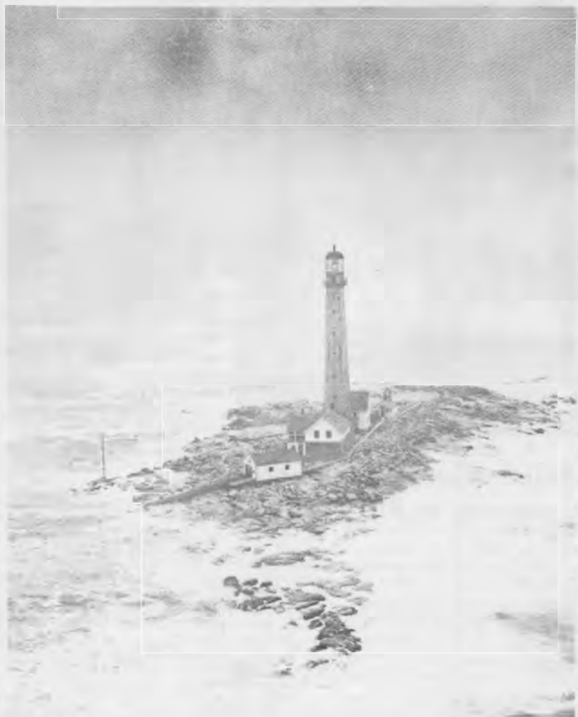
Boon Island Light Station, Maine. (U.S.Coast Guard Official Photo.)
